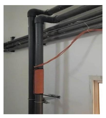
Around 40 coils are done on the inlet pipe of RO plant 2 Installation Date: 10<sup>th</sup> September 2020
