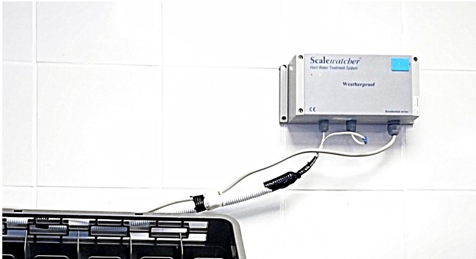
**SW Commercial Model installed in the 2" inlet pipe of the dishwasher system with 1 set of coil of 40 loops**
