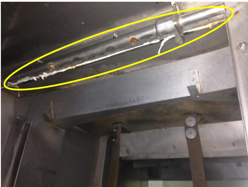
6<sup>th</sup> Nov 2016, the scaling patches are being clearly removed at the bol nut edging them and at the sprayer as well giving it a brand new look
