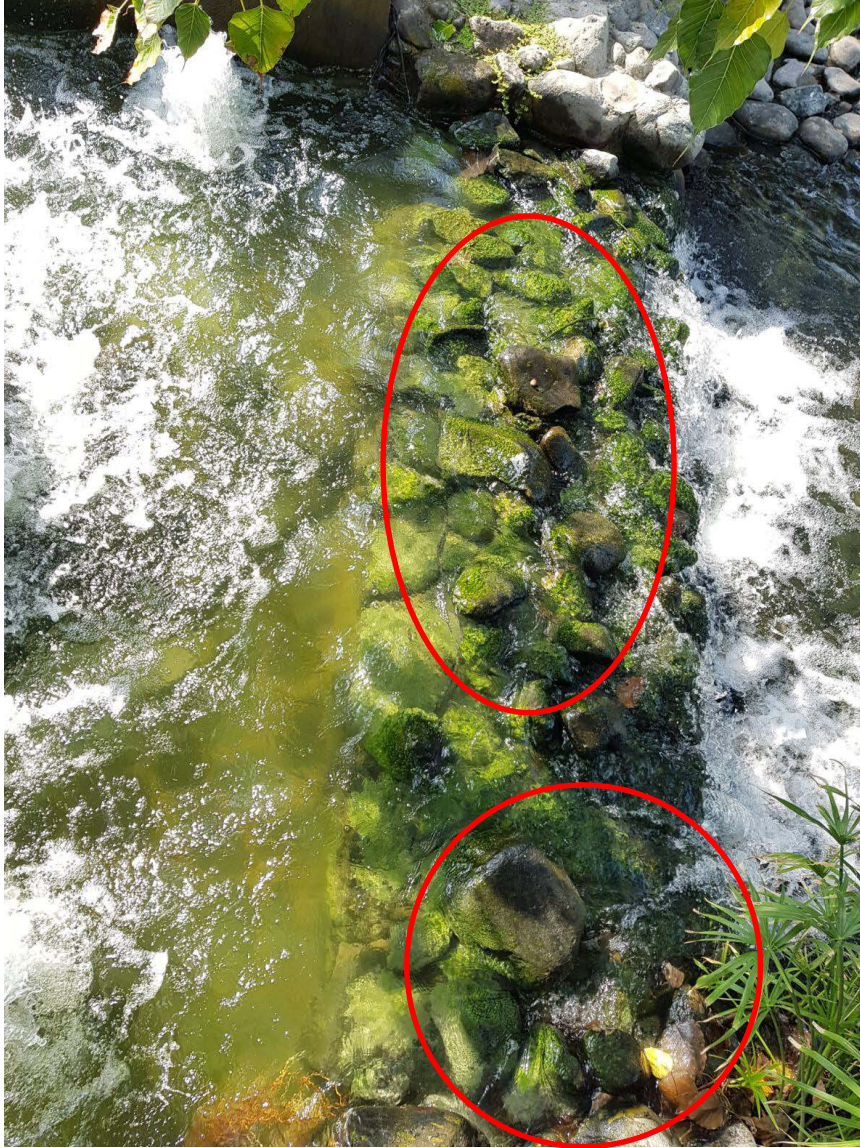
Before Installation 27 th November 2017
