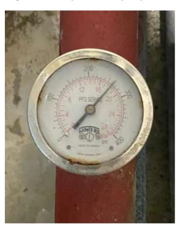
After treatment (week 3), the image clearly shows that the pressure in guage has dropped due to melting of scaling in the pipeline
