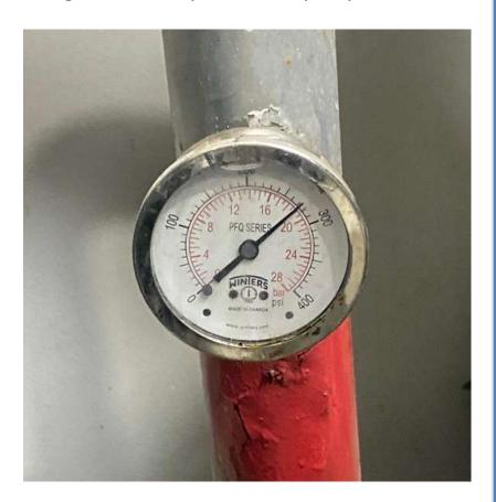
After treatment (week 3), the image clearly shows that the pressure in guage has dropped due to melting of scaling in the pipeline
