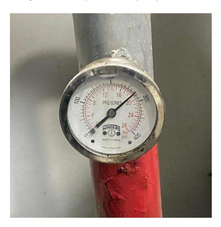
After treatment (week 1), the image clearly shows that the pressure in guage has dropped due to melting of scaling in the pipeline
