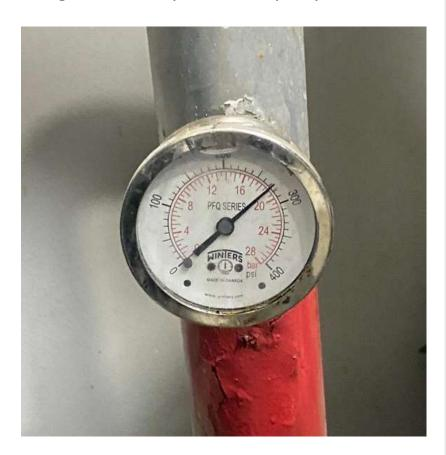
After treatment (week 4), the image clearly shows that the pressure in guage has dropped due to melting of scaling in the pipeline
