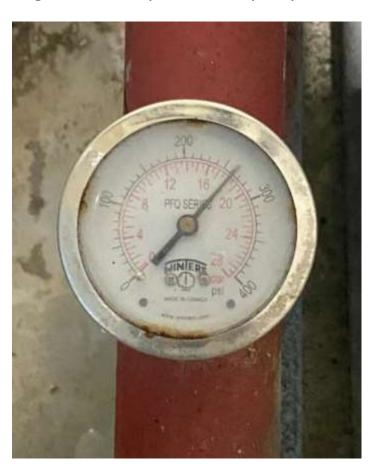
After treatment (week 1), the image clearly shows that the pressure in guage has dropped due to melting of scaling in the pipeline
